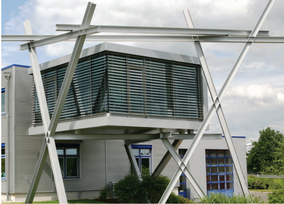
This building in Erbdorf, Germany features an exterior venetian blind system.
