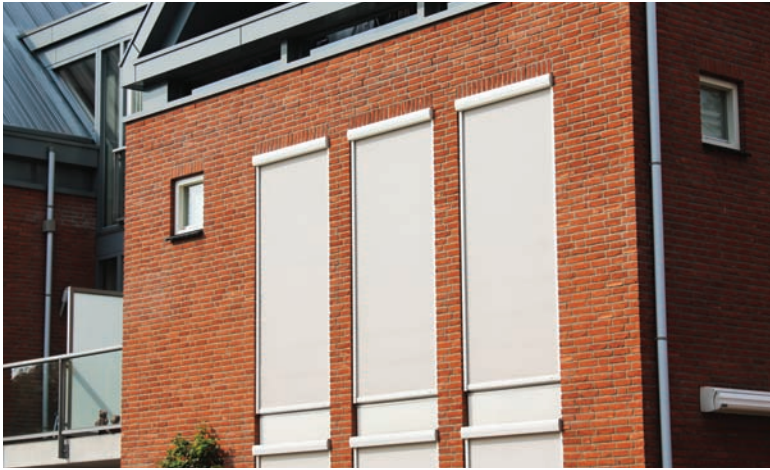
This installation in Holland features solid-screen, 'zip' system installation.
